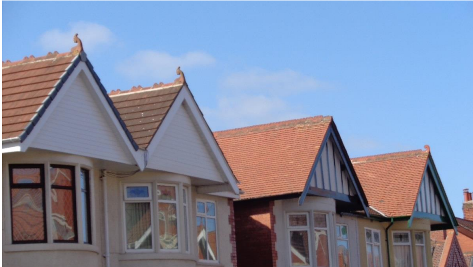
Original half-timbered gables to the right, upvc clad gables to the left
